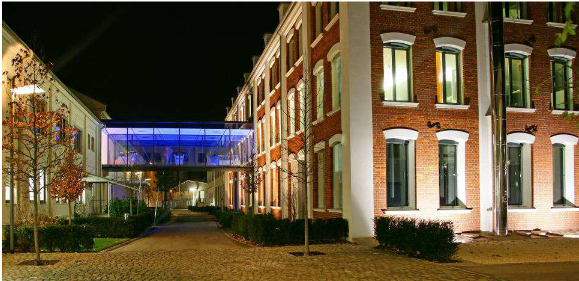
Abb. 8: The historical buildings retrofit to passive house for company Fronius in Wels Fotos: PAUAT Architekten/Luttenberger
