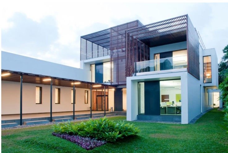
Passivhausprojekt in subtropischen Klimate: New Austrian Embassy Jakarta, Generalplaner/Lead architect: pos architecture Vienna, Client/ Bauherr: BMEIA/ Austrian Foreign Ministry, Foto: TimX.C.
